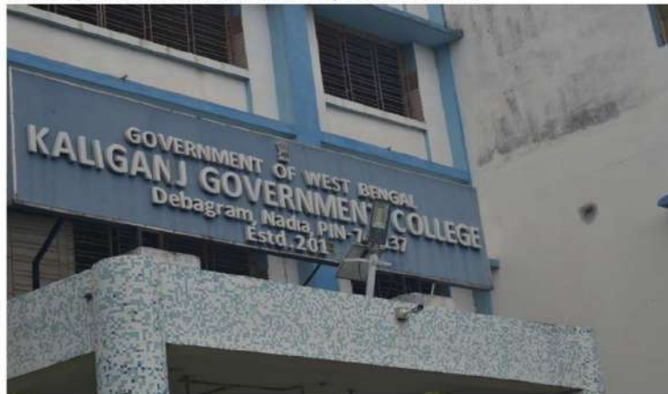
Picture of Solar Light installed at the entrance of the building
