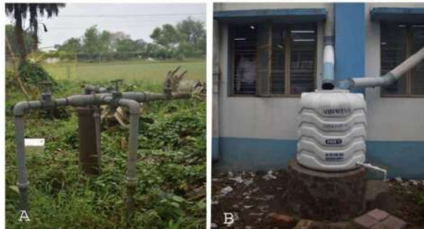
separate soak-pit to avoid direct contamination. To avoid arsenic, lead and Plate: A. Borewell near ground, B. Rainwater Harvesting System
